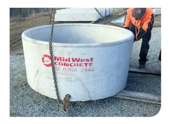
Lift and position the trough at its final location. Ensure it is stable, level and ready for use.
