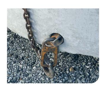
Ensure the clutches are correctly secured to the lifting hook and are not twisted or tangled.
