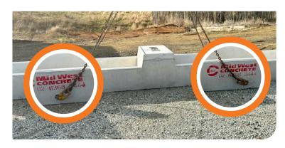
Lift and position the trough at its final location, whether at ground level or raised. Ensure it is stable, level and ready for use.
