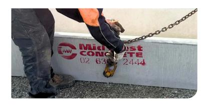
Check that all lifting clutches are securely attached and the chains are not twisted.
