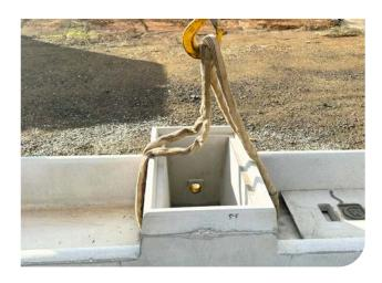
Lift and position the trough at its final location, whether at ground level or raised. Ensure it is stable, level and ready for use.
